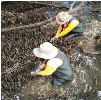
Mangrove drainage channels are hand-cleared to maintain tidal flows and thus prevent ponding and dieback
