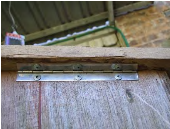
Figure 6. Hinge screwed into side and up under lid using good quality screws
