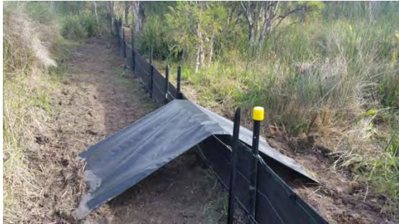
Figure 3 The second Gambusia fence (600mm high) with shade cloth ramp.
