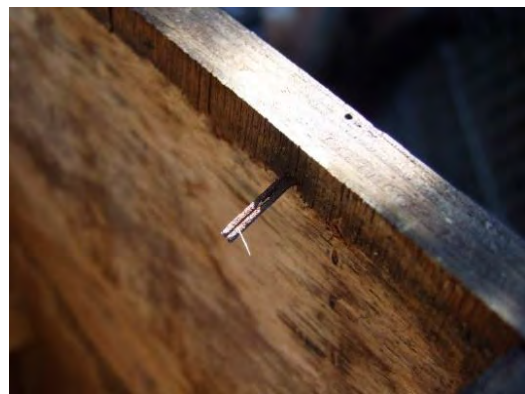
Figure 1. A staple (shown here) and nails do not hold as well as good quality screws
