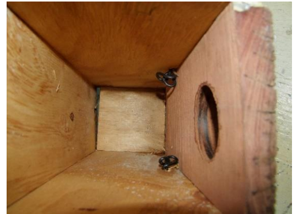
Figure 9. Wire knots inside box stops the wire from pulling out
