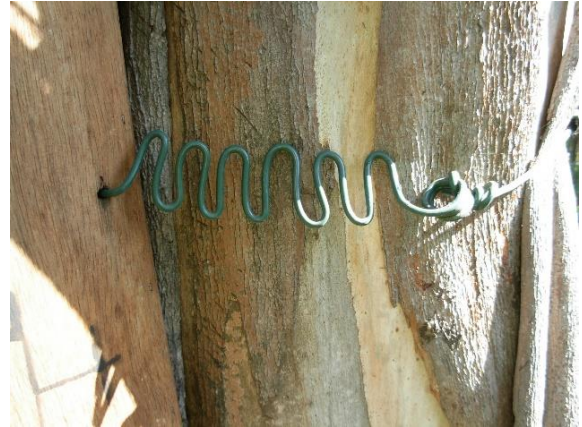
Figure 8. Expanding zig zag Habisure attachment
