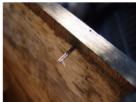
Figure 1. A staple (shown here) and nails do not hold as well as good quality screws
